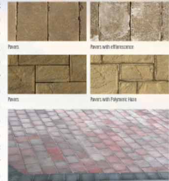
Efflorescence emerged from pores within a magnified area of a concrete paver. The calcium has been carried to the surface by water.
